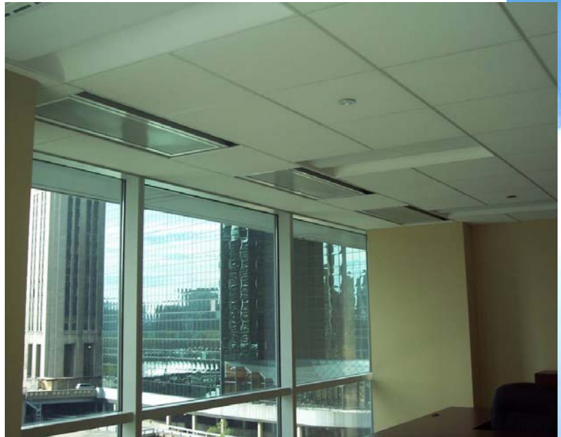
ACB50 incorporates I-way supply air discharge with a one piece perforated return air grille and single horizontal secondary cooling coil
