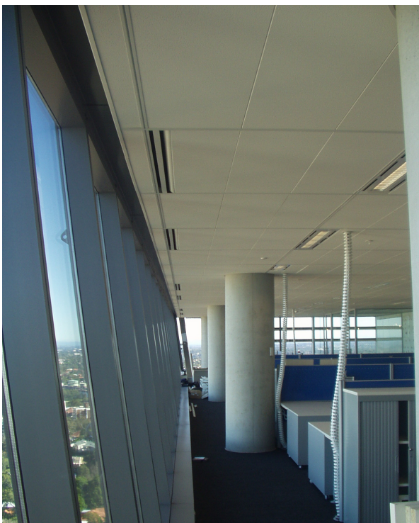
Typical Perimeter Inffusers
