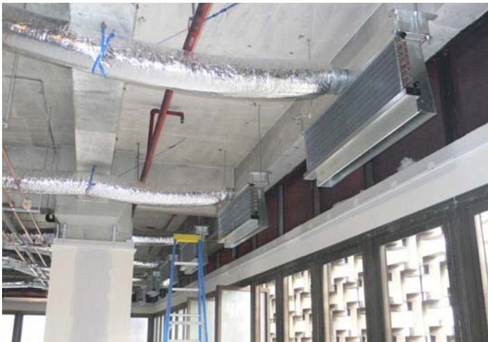
CM10 Units Installed at Perimeter
